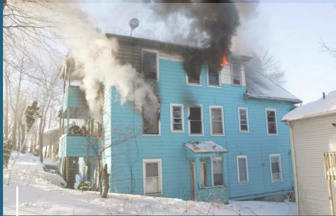
A house fire
