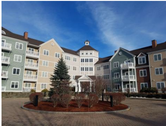
Maritime Landing, Newburyport
