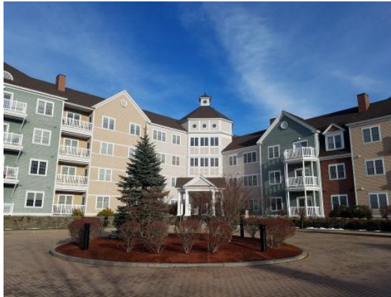
Maritime Landing, Newburyport
